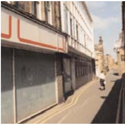
Mercury Row – poor frontage
