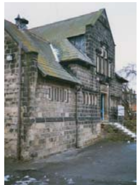
Former National Infants' School, Wharfe Street
