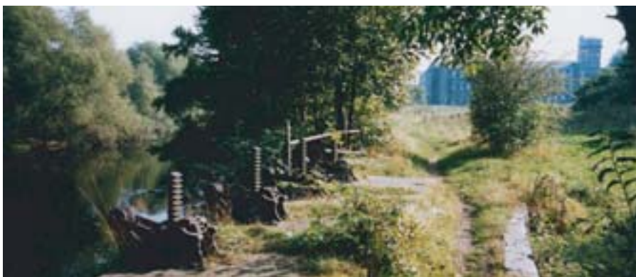
Otley Mills sluice gates
