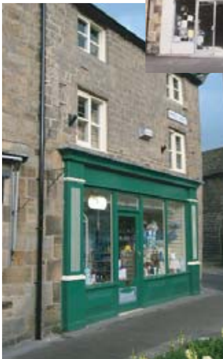
1 Bridge Street – shopfront restoration
