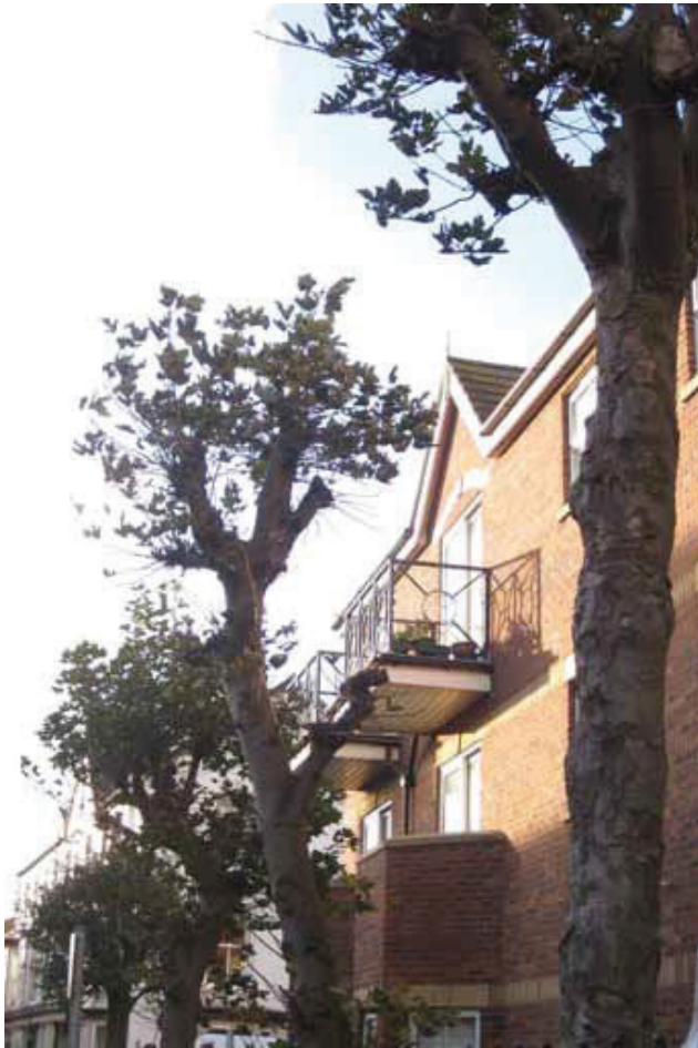
Poor relationship: Maple trees too close to flats necessitate continuous harsh pruning and disfigurement to reduce the canopy sizes
