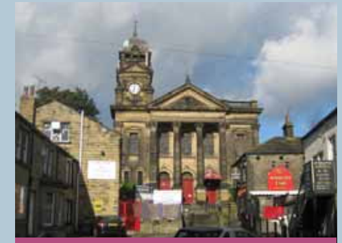
The Trinity Methodist Chapel is a key landmark and point of orientation around Pudsey.
