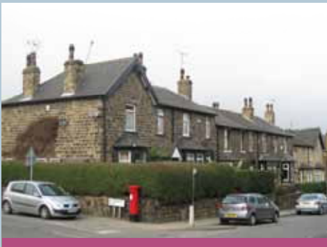
Strong two-storey frontage along Richardshaw Lane
