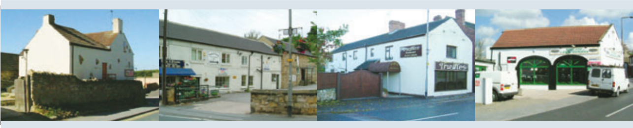
No. 5 Leeds Road, currently a Balti Restaurant, dates from the 17th century
