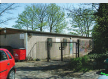
Kippax Kabin, a small pre-fabricated building is the only specific amenity for youth. A better, bigger, permanent facility is recommended for the youth of Kippax.
