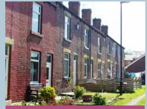
Brick terrace with stone detailing, Clayton Street
