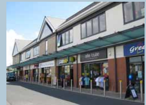
Integrating the new development with the historic town is one of Rothwell's biggest challenges
