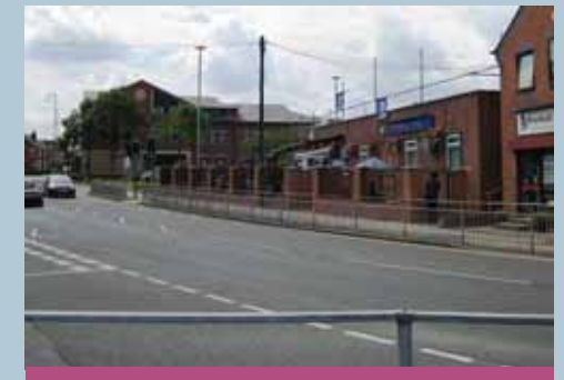
Some public realm treatments detract from the quality of the conservation area and offer an opportunity for enhancement, Marsh Street
