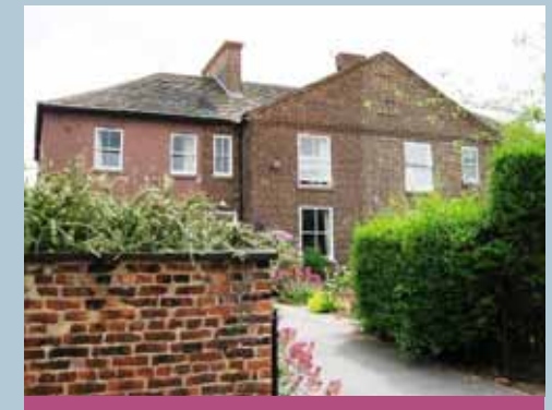
Prospect House was built as the Parish Poor House in 1772 on reclaimed marshland
