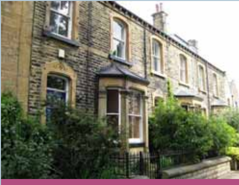
Low level stone walls with copings, iron railings and gates are important to the character of The Paddock
