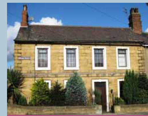
Prestigious stone-built listed building, 2 Marsh Street
