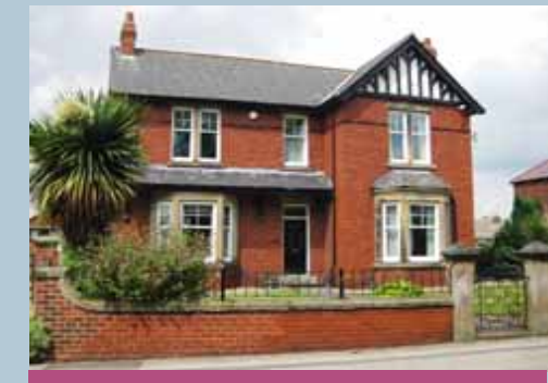
Red brick Edwardian villas are a distinctive feature of the town; this example at Royds Lane
