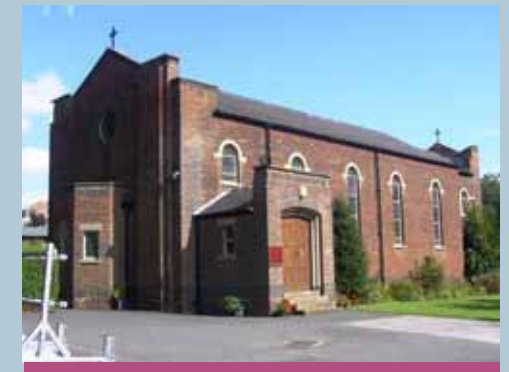
St Mary's Catholic Church is a local landmark building
