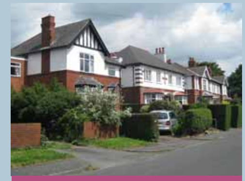
Distinctive early 20th century suburban development, Churchfield Road
