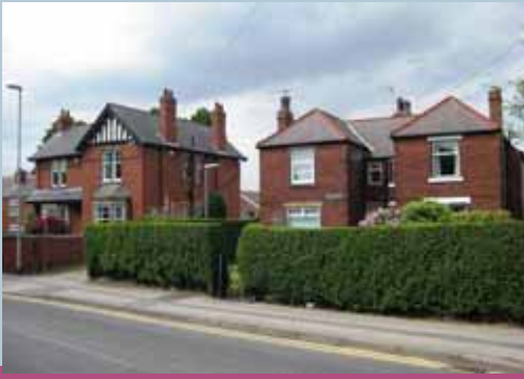
Brick boundary walls and hedges are important boundary treatments, Royds Lane
