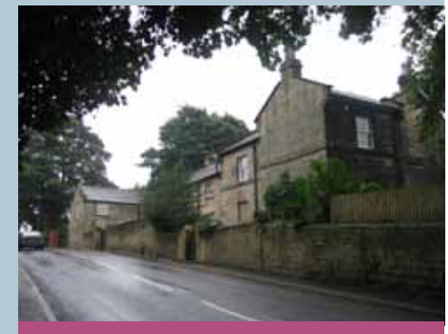
19th century structure on Church Hill
