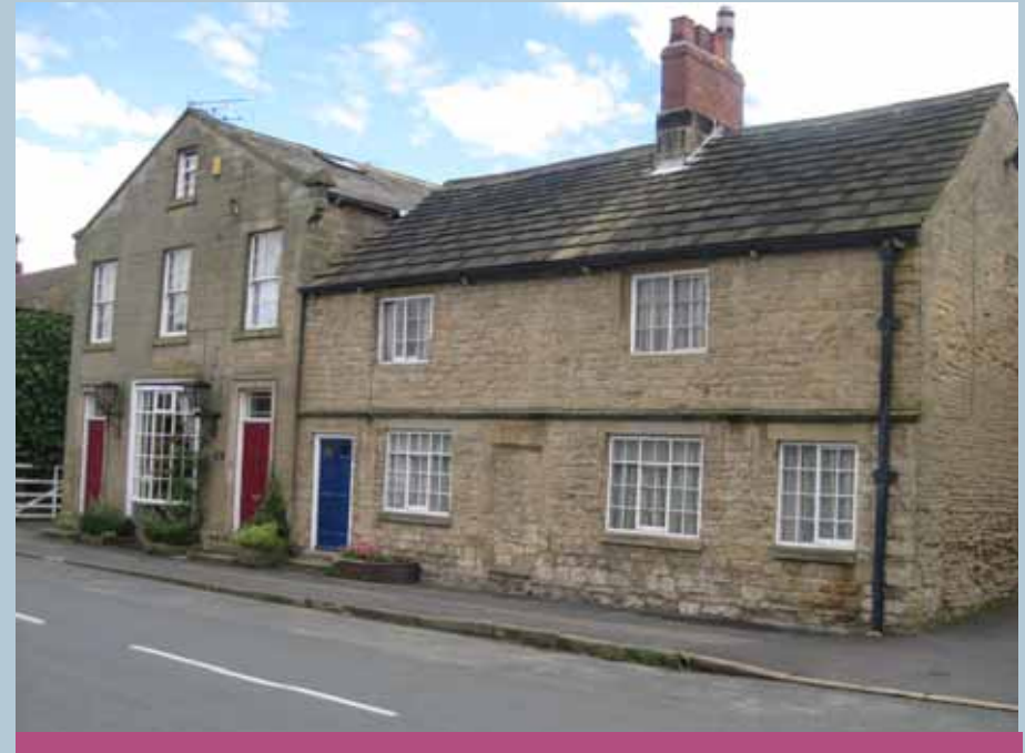
Traditional detailing can be seen to add character to historic structures, such as the stone surrounds on the windows, cast iron rain water good, and traditional windows.
