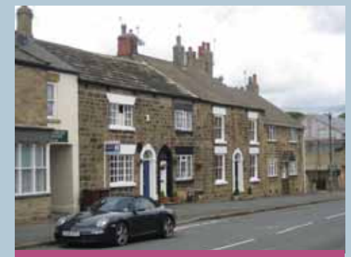
Architectural detailing is a key characteristic of much of Main Street
