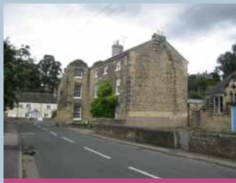
Historic architecture and boundary walls on Church View
