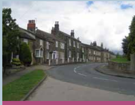
The sweeping road bend on entering Main Street
