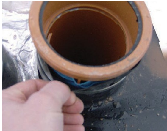
Figure A4.28 Bead of double sided butyl tape provided between interfaces of ID top hat and OD service pipe. When compressed with jubilee clip, forms an effective seal (courtesy Smith Grant)
