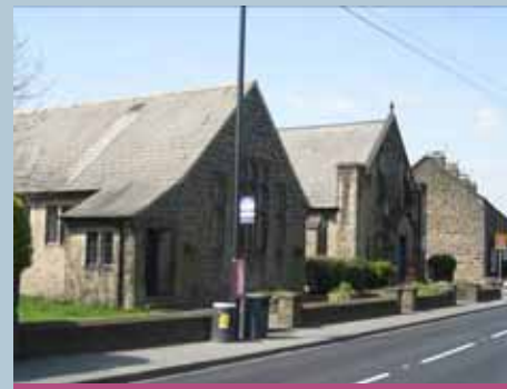
Ecclesiastical buildings located within central Pool are one element of the varied architectural palette which is present within the Pool conservation area.
