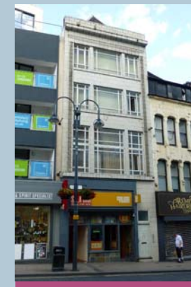
Early 20th century white faience building south end of New Briggate
