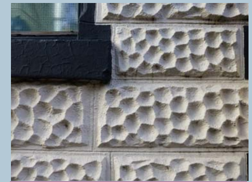
Nash's stucco intended to resemble rock-faced rusticated ashlar
