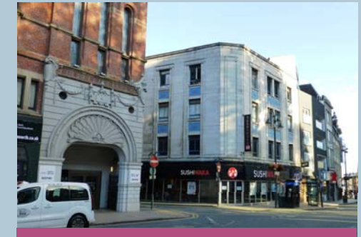
Early 20th century building at the southern end of New Briggate on the site of the earlier vicarage
