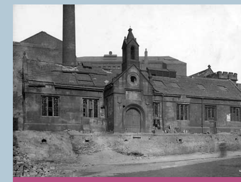
Harrison's Grammar School of 1624, previously on Vicar Lane, demolished c1900 ©Thoresby Society
