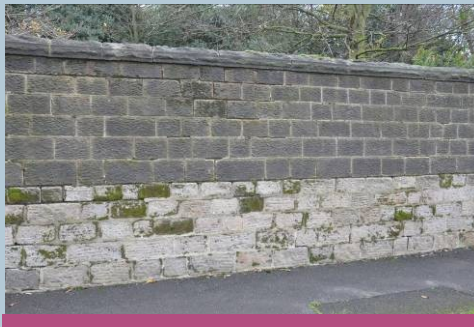
High boundary wall on Apperley Lane, raised in the 19th century.
