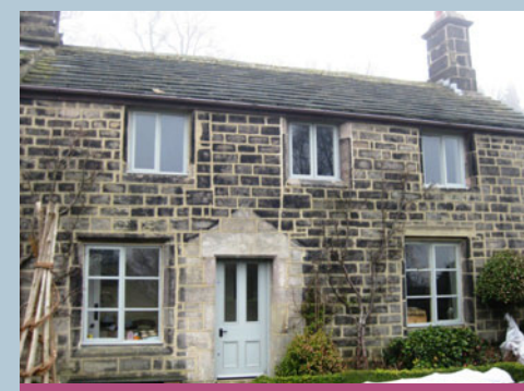
Grade II listed Dove Cottage (incorporating Buckstone Cottage) dates from the late 17th century.
