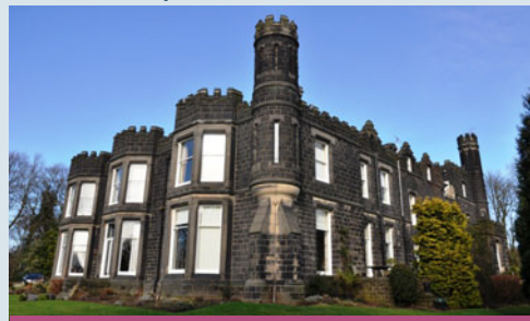
Grade II Buckstone Hall, 1884. Architects, Lockwood & Mawson.
