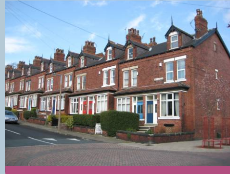
Methley Terrace. Note the slate-hung dormers with bargeboards and finials, decorative chimney pots and paired first floor windows.
