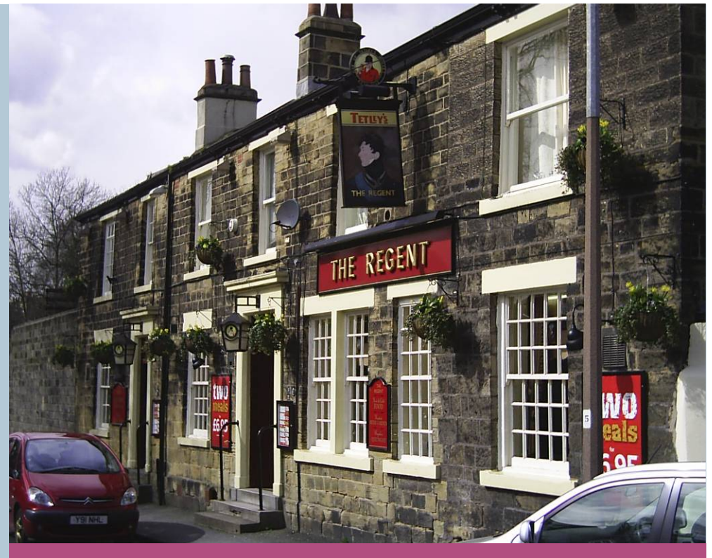
The Regent Inn, Regent Street, built in the early 19th century, which has been a pub since at least the 1840s.
