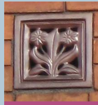
An air brick manufactured by the Leeds Fireclay Company of Burmantofts, an example of the decorative detailing to be found in the Methleys.
