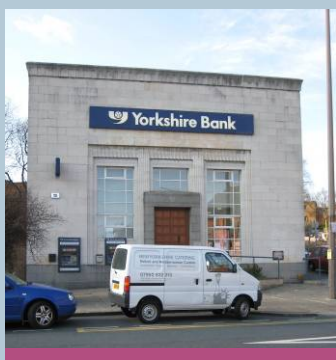
Yorkshire Penny Bank building, Stainbeck Corner. Built in the late 1930s, this small building is a good example of the stripped-down Classicism of Modern architecture between the wars.
