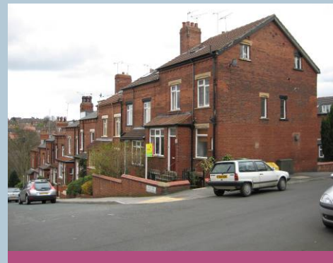
Pasture Crescent, a Type 3 back-to-back built between 1920 and 1934. Note the external basement access to the indoor lavatory and the very small larder window on the front elevation.
