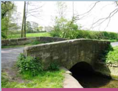
Firgreen Bridge over Carr Beck looking back toward The Willows
