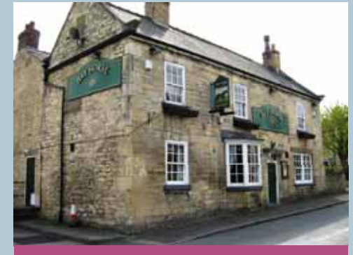
The Bay Horse; the side gable shows the building has been extensively altered. The current façade is clearly a later addition.
