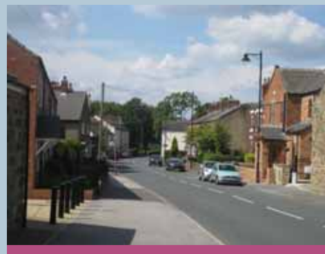
The conservation area is focussed around the linear development of the historic village along Main Street
