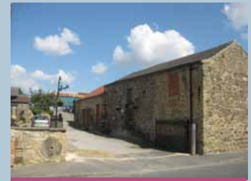
Green Lodge Farm contains historic outbuildings which were once characteristic of Scholes.
