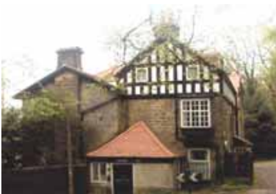
'Hillside', former home of architect Sidney Kitson.
