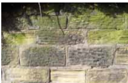
Hand-hewn local stone is the main building material.
