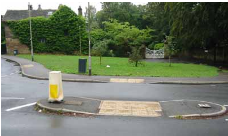
This important green space at the heart of Gledhow has been harmed by visually unsympathetic highway works.
