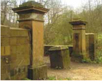
Carriage drive gates to Gledhow Hall.
