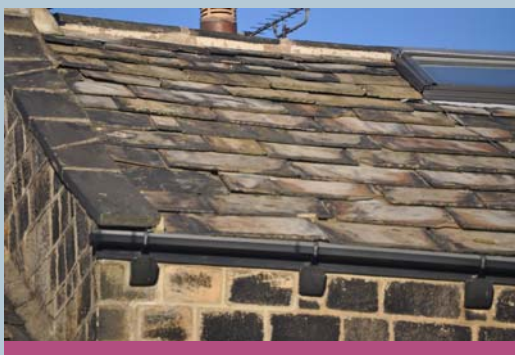
Characteristic stone slate roof. Note the dentilled eaves.
