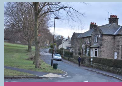
Park Road encompasses elements of shared surface and is important to retain as a minor road in order to preserve the character of the moor area.
