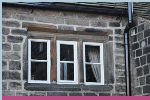
The mullions and timber window frames of character area 5.
