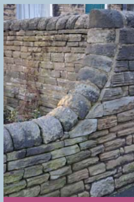
Characteristic sandstone walls and coping stones.
