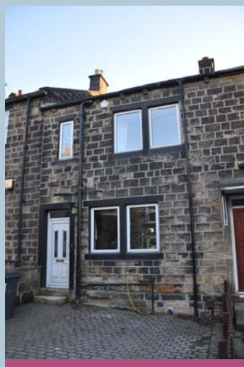
Evidence of the old weavers industry in the larger first floor window to this mid terrace house.
