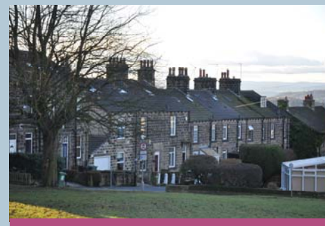
The characteristic rows of terrace cottages.
