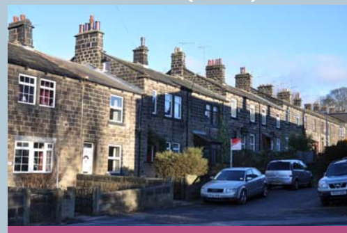
The characteristic lines of sooted stone terraces. Note the extensive chimneys, low front garden walls and some remaining mullioned windows.
