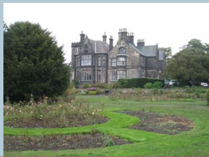
Micklefield House provides an element of hierarchy to Little Moor and is an important positive building.
