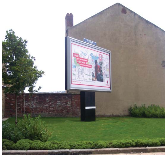
▲ Previously derelict site in City Centre commercial area improved by attractive and well maintained landscaping
