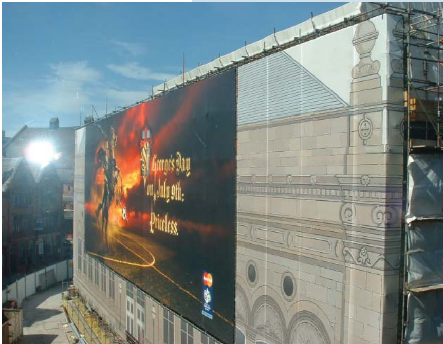
▲ A building wrap on a scaffolded listed building
