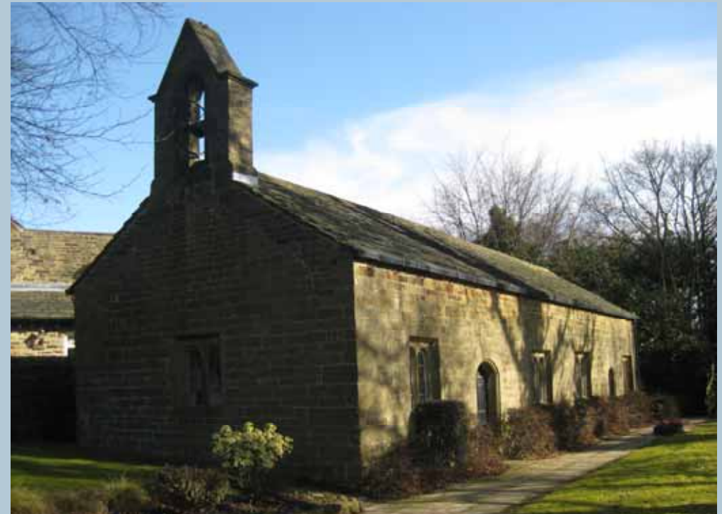
The Grade I listed Puritan Chapel is not only of immense architectural and historic importance, it is also a key element in the development of Bramhope, the Dyneley estate and Bramhope Hall (now demolished).
