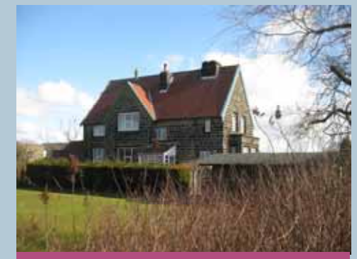
The Robert Craven Memorial Hall is one of the few buildings dating from the 19 th century in Bramhope
