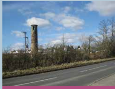
The listed siting tower (outside the conservation area) is a key reminder to 19 th century construction of the Bramhope railway tunnel
