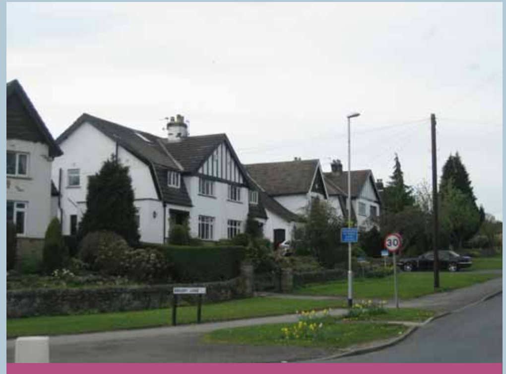
The wide grass verges and front gardens and walls associated with the 20th century housing in Bramhope are important features in establishing an informal character in the Bramhope Conservation Area.
