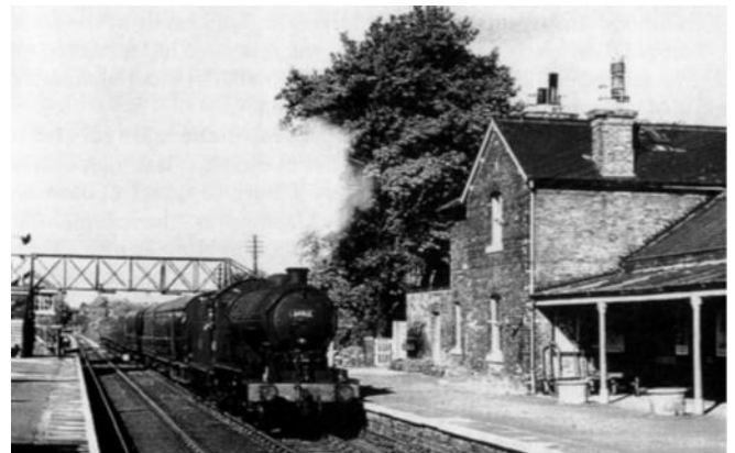
Photo 8.1 Collingham Bridge Station
