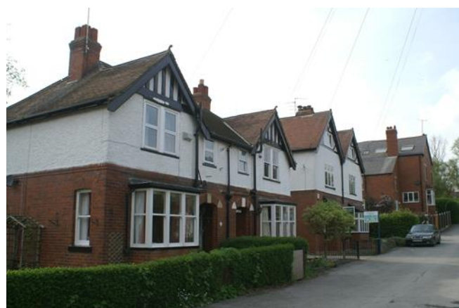
Photo 14.2 Forward facing gables
