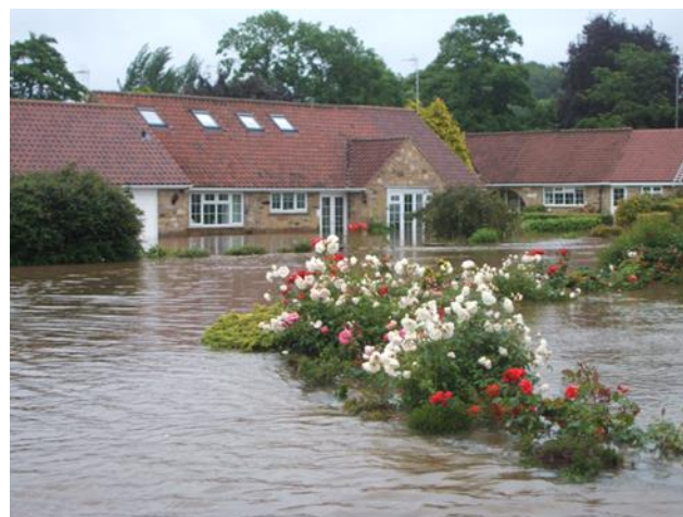
Photo 16.1 Flood The Close (Millbeck Green) 2007
