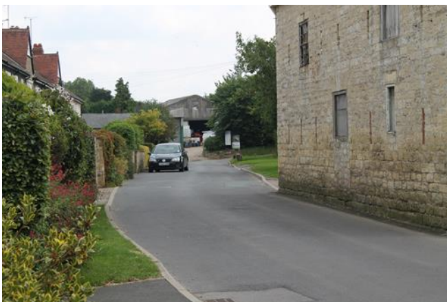
Photo 23.1 School Lane intermittent footway
