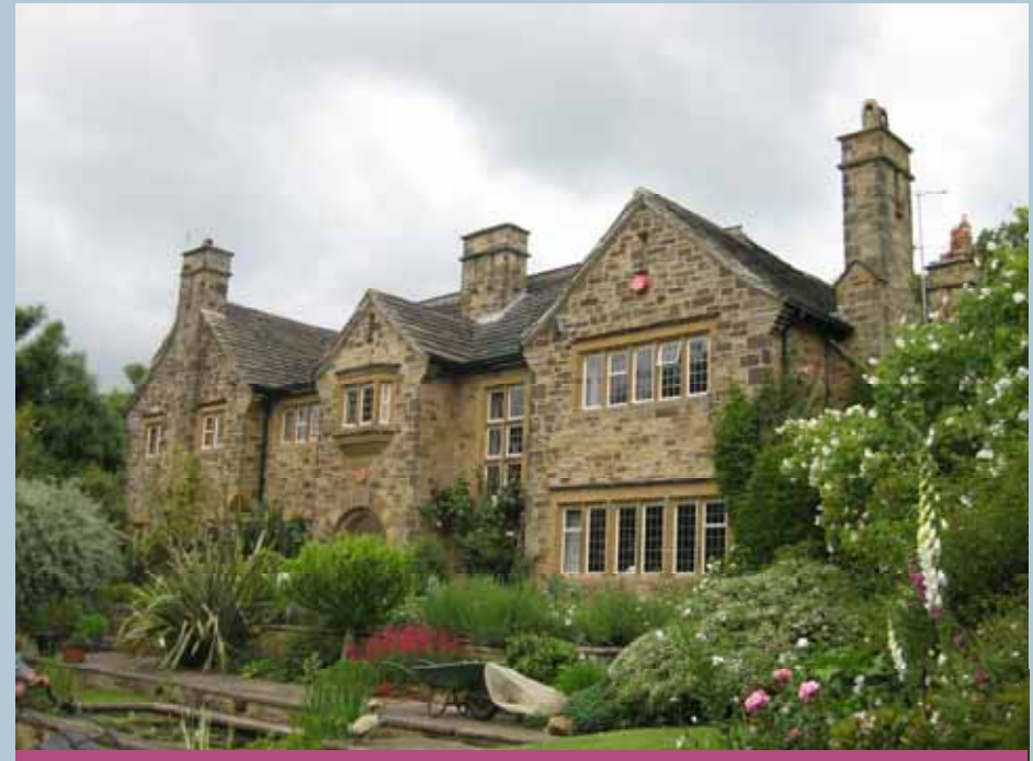
1920s structures such as Hard Gap present one aspect of the variation of the style of architecture which is present within the Linton Conservation Area.
