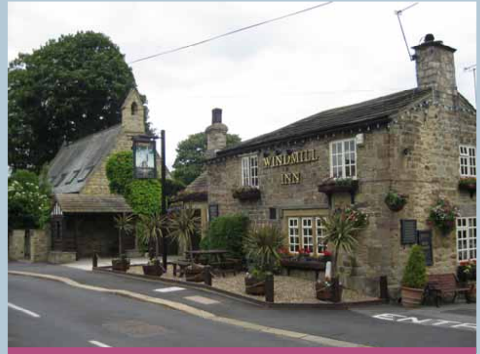
The Windmill Inn and the converted church building are both important buildings to the conservation area. The traditional appearance and maintenance of historic details helps establish the character and appearance of the conservation area.
