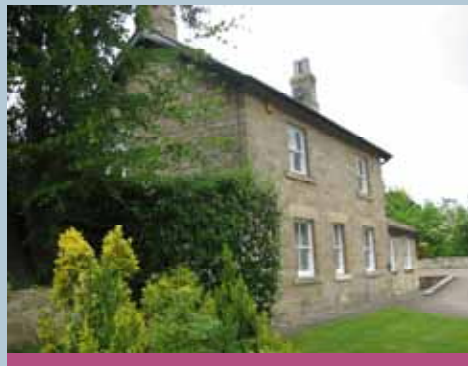
Exposed coursed natural stone is the predominant walling material within the conservation area.
