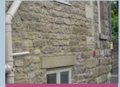
Regularly coursed natural stone should be retained as the predominant building material.
