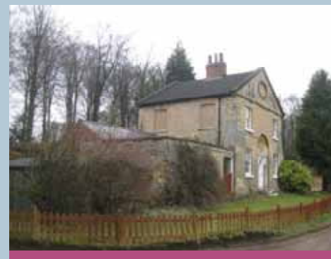
Parlington Lane Cottage is an imposing Georgian building constructed along Parlington Lane.
