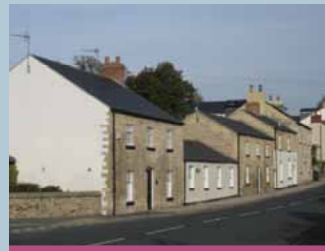
A mix of render and natural stone provide variation in the domestic properties appearance within the conservation area.
