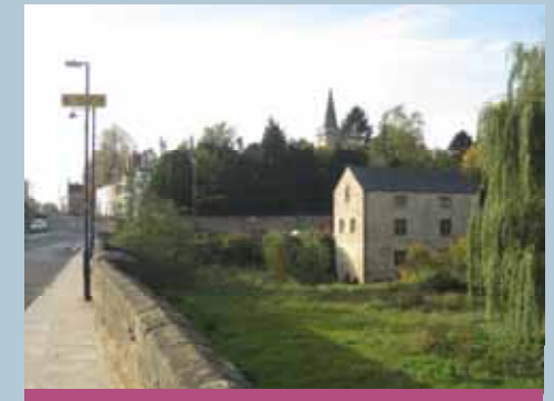
The former water-powered corn mill may have its origins in the 14th century.
