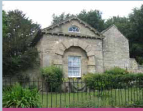
The Hookmoor Lodges are a focal point at the southern access into the conservation area
