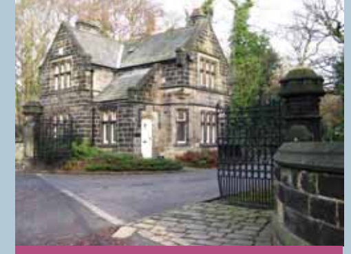
Impressive gateways with lodges are the public face of the mansions, Weetwood Hall
