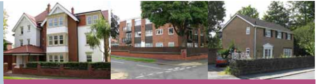
Recent development has been of mixed success in terms of responding positively to the character of the area
