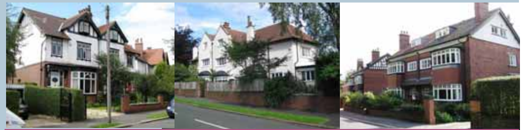
Buildings are large, generally of three storeys with dormer windows
