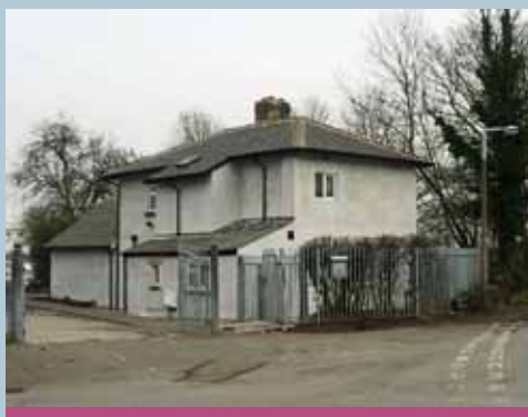
Spen Lane Cottage (now The Cottage ), originally an isolated roadside cottage set within fields, shown on a map of 1839
