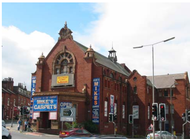
The condition of 2 Branch Road is a blight on the conservation area
