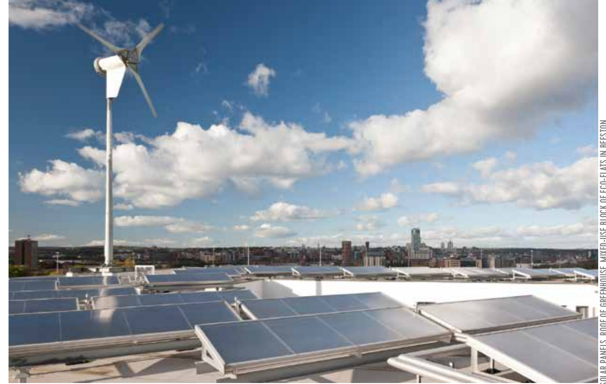
SOLAR PANELS, ROOF OF GREENHOUSE, MIXED-USE BLOCK OF ECO-FLATS IN BEESTON
