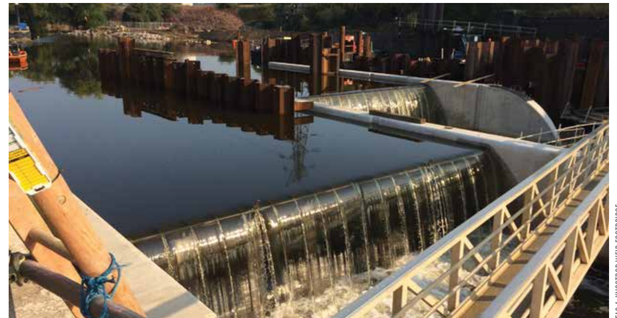
FAS 1: KNOSTROP WEIR FOOTBRIDGE
