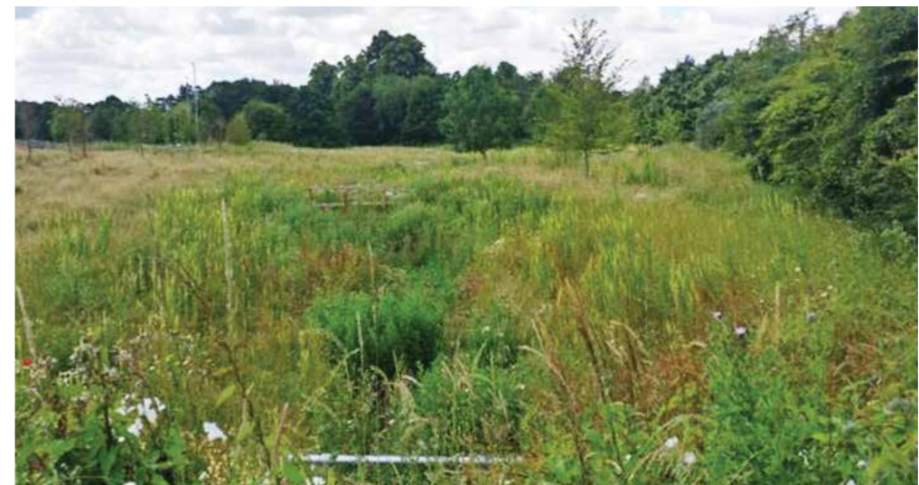
AFTER: WYBE BECK VALLEY IMPROVEMENT PROGRAMME, THE ARTHURS REIN SCHEME CONSISTED OF SWAPPING A DRAINAGE PIPE COLLECTING SURFACE WATER IN THE AREA AND OUTFALLING INTO WYBE BECK, INTO AN OPEN WATERCOURSE
