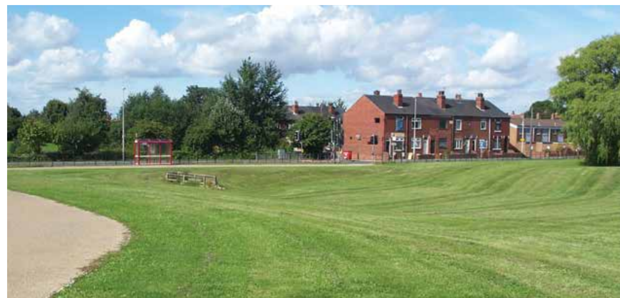
SUSTAINABLE DRAINAGE AT ALLESTON BYWATER
