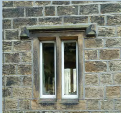
Mullion and drip mould characteristic of the 17/18th century
