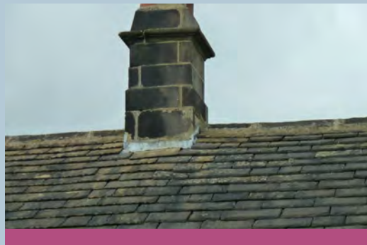
Characteristic stone slate roof. And ornate chimney.
