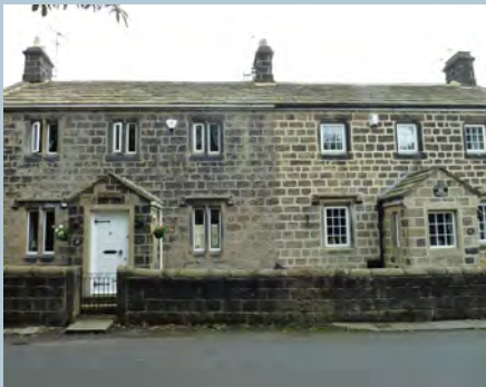
Properties on Gill Lane. Note the removal of mullions on the right hand property.
