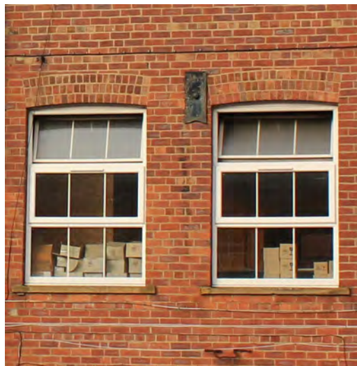
uPVC windows on Mabgate Mills
