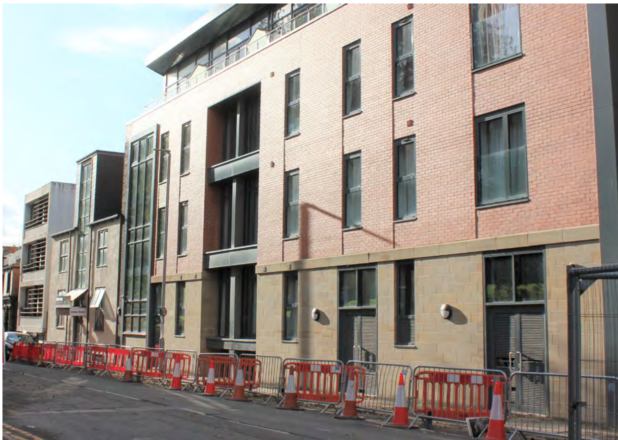
Inactive street frontages with poorly designed ground floors in new development in Mabgate
