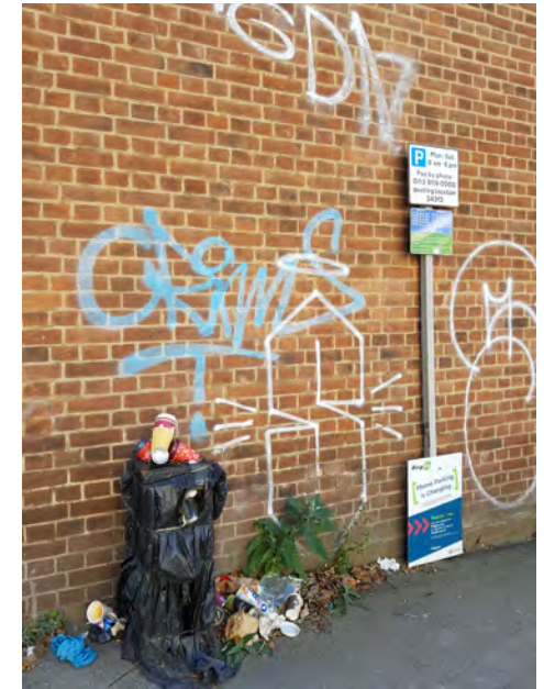
Rubbish, graffiti and poor public realm within the Regent Street character area
