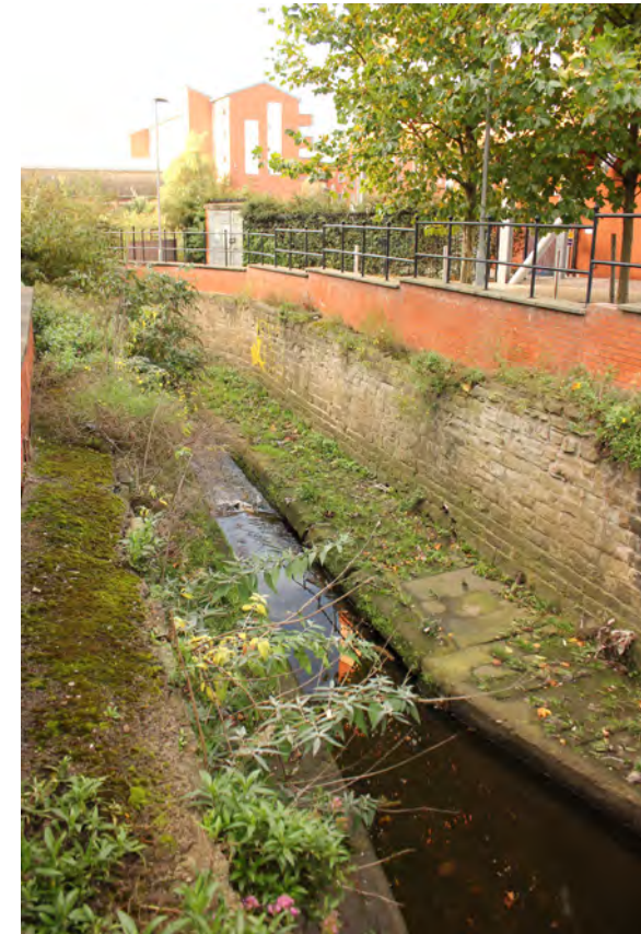
Looking south-west from Skinner Lane bridge
