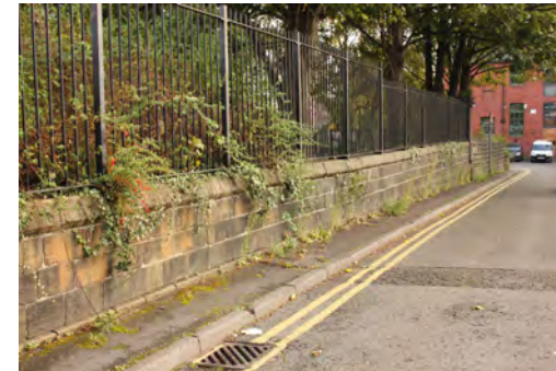
Stone wall St Mary's Street
