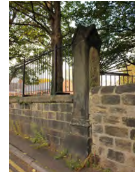
Stone wall St Mary's Street
