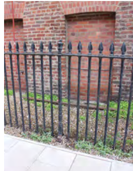
Railings - Mabgate Mills
