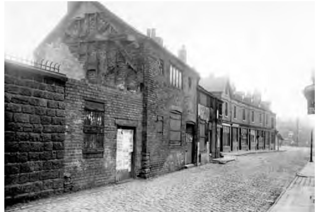
The corner of Mabgate and St Mary's Street. Mabgate, 1919. Note the timber framing on the gable end in the foreground of the dilapidated house to the right. (Leeds Library & Information Services)
