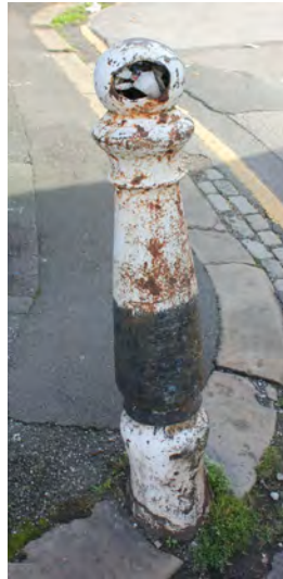
Bollard, Millwright Street
