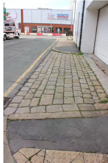
Early 20th century stone setts and kerbs, Millwright Street
