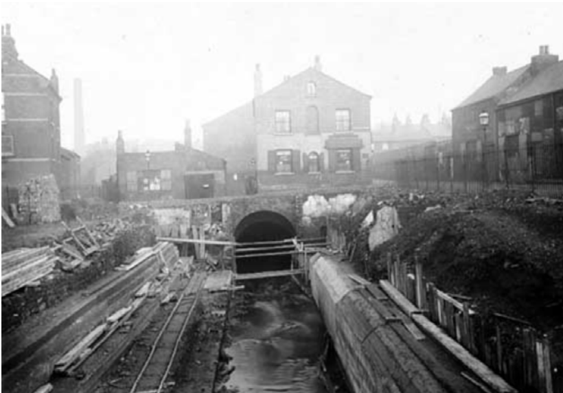
The culverting of the Mabgate Beck in Mabgate 1914 (Leeds Library & Information Services)
