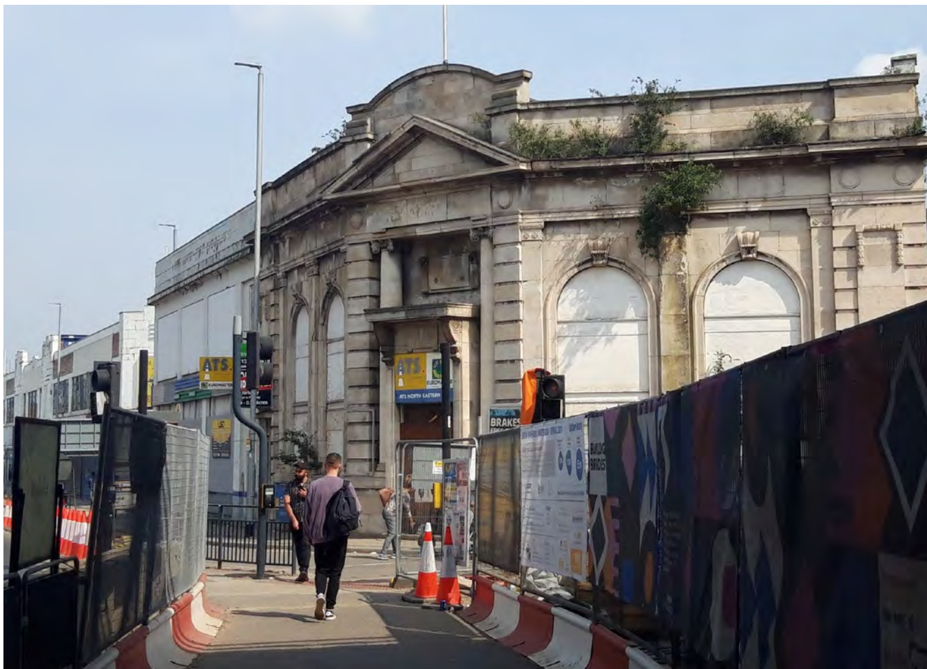
The former Yorkshire Bank; vacant and roofless
