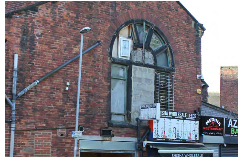
Altered chapel window, Mushroom Street
