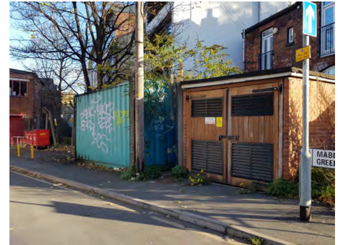
Electricity substation, signage, telegraph pole, bins and storage container, Mabgate Green
