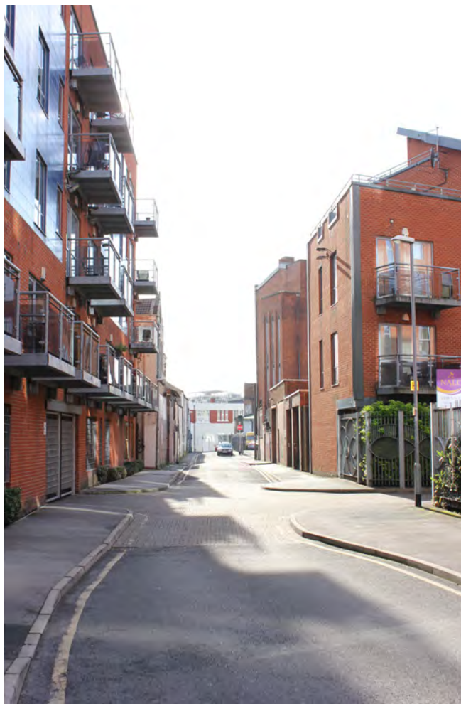
Millwright Street new development
