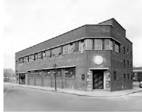
The ATS building on Mabgate 1938 former premises of the British United Shoe Machinery Company. (Leeds Library & Information Services)
