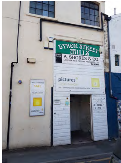
Inappropriate alteration at Byron Street Mills
