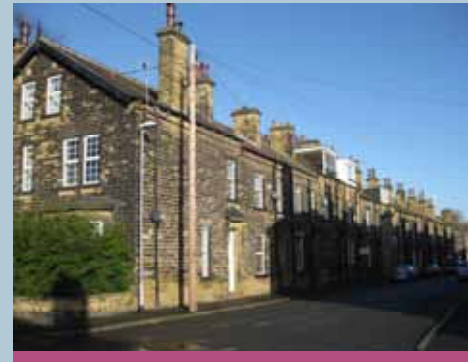
Locally quarried millstone grit provides the bulk of the building material within Bramley.
