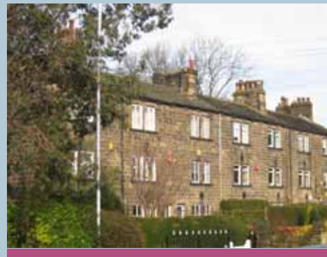
Terrace rows, such as at Moorfields are an example of the high quality architecture that still exists within the rest of the character area.
