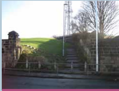
Opening in the boundary wall of the park on Broad Lane provide access into the park at various intervals
