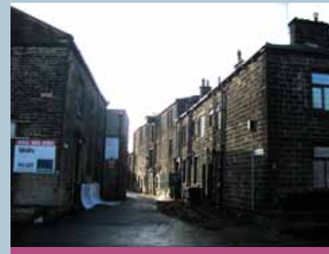
Very little remains of Bramley's industrial development. An exception is Haley's Yard off Upper Town Street
