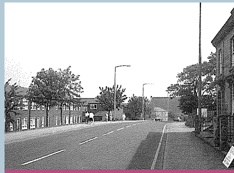
By 1991 the character shown here had changed dramatically. This image is taken from the same location as the image above (both images taken from Silson's Bramley Half a Century of Change )
