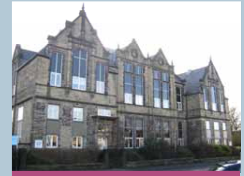
Municipal architecture (both existing and former) such as the converted school on Broad Lane highlight Bramley's 19th century wealth.
