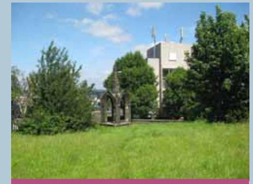
Remains of a part of the former medieval church of St Margaret, within the land adjacent to the existing St Peter's Church
