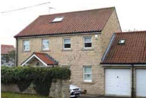
◀ Contemporary additions have used traditional materials and details found on older properties, such as window proportions, head and sill styles and pitched canopies over the doors. Garages and taller boundary treatments assist in absorbing the car from the street scene. Chimneys are not used which distinguish new dwellings from old, but do not contribute as strongly to rhythm of street.
