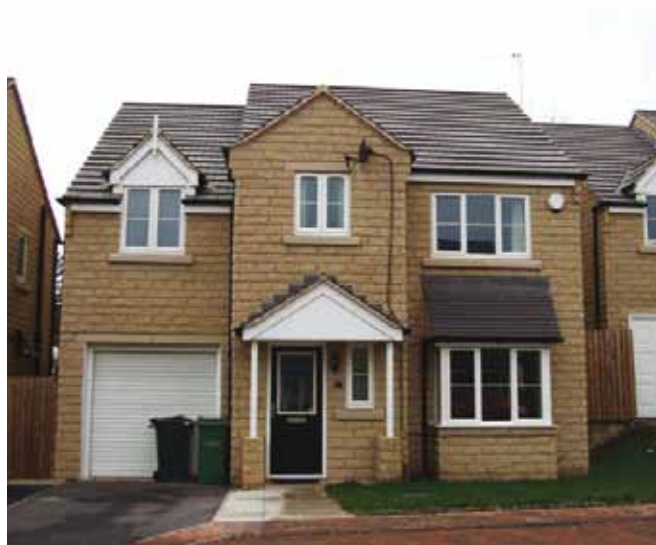
The small bay window and the canopy are very simple additions which do not detract from the appearance of the main dwelling.
