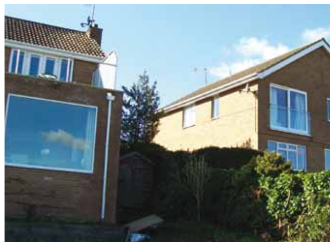
Where balconies, terraces or decking project out from the house a solid screen to the side will be needed to prevent overlooking of neighbours. Juliet balconies do not allow a person to step out and so no screen is needed.
