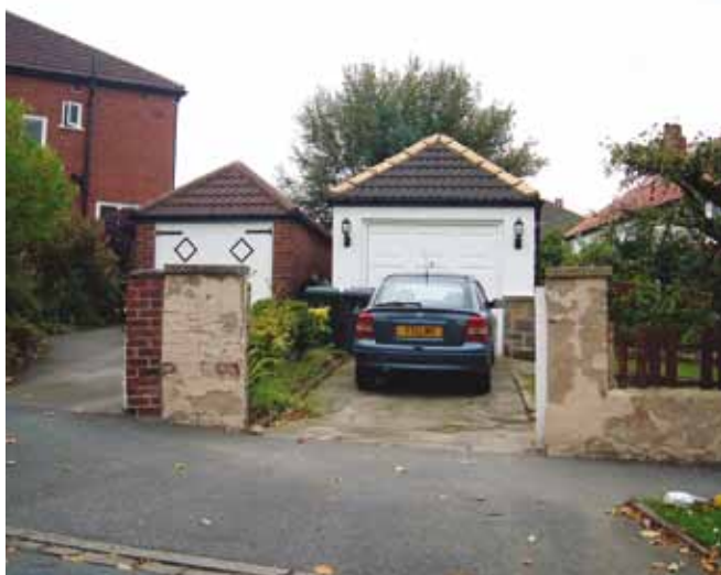
This garage has a simple shape and form and allows plenty of room to its front to park an additional car. It is important that cars do not overhang onto the footpath and also allow the doors and the boot to be opened without blocking the footpath.
