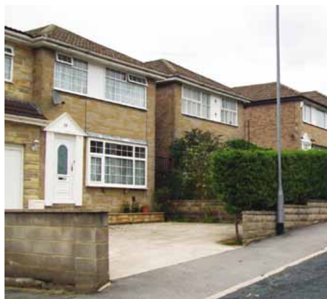
Large areas of tarmac or concrete to the front of properties can be very hard and stark. They also create surface water run-off and can contribute to flooding. Areas of vegetation to the front boundary help to soften the appearance of the parking area and can also help drainage.
