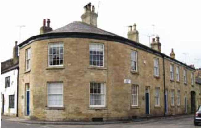
The curved frontage of these buildings is a unique feature and creates an interesting streetscape. Other details such as the window forms, doors and chimneys contribute to the character of the properties and all such details are important.
