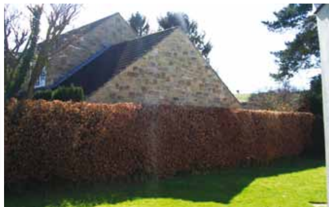
Care should be taken to ensure that extensions do not overshadow or overdominate neighbouring gardens and windows.
